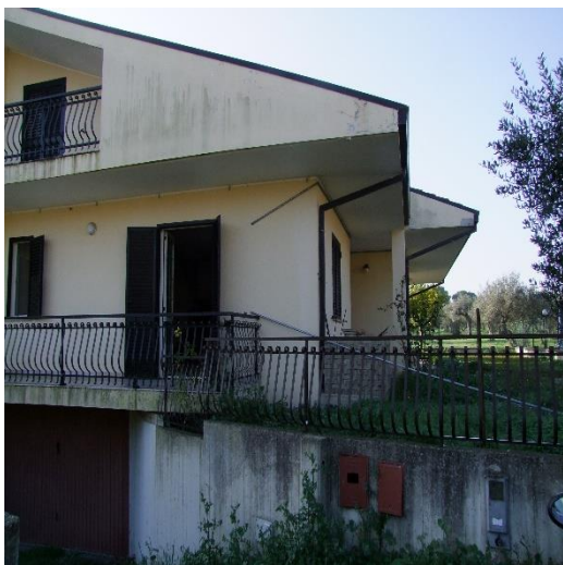
FOTO 45: ACCESSO AL GARAGE AL PIANO SEMINTERRATO, P.LLA 4259 SUB. 2 (B.C.N.C.)
