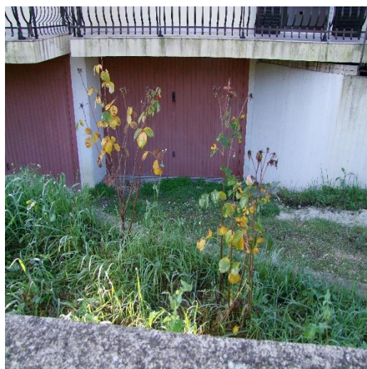
FOTO 44: ACCESSO AL GARAGE AL PIANO SEMINTERRATO, P.LLA 4259 SUB. 2 (B.C.N.C.)
